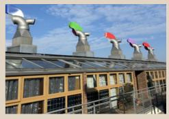
The development's most striking feature is the colourful wind cowls that orient themselves towards the wind, naturally ventilating spaces through a heat exchange.
